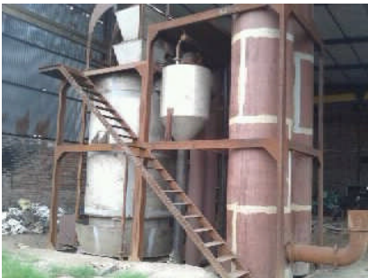
CHAMCO 1 MW Gasification under Construction
